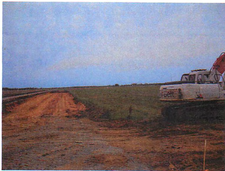
View Southeast Rail siding grading located on left
